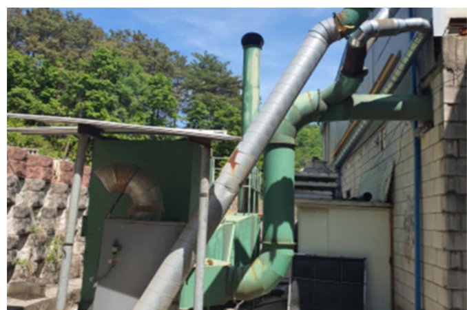
Existing VOC's removal facility(30m 3 )
